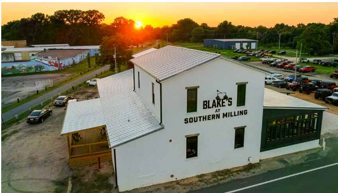
Sunset brings another busy night for the crew at Blake's at Southern Milling.
